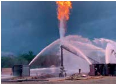
Capping BOP stack successfully placed over the well head on 17 August 2020
