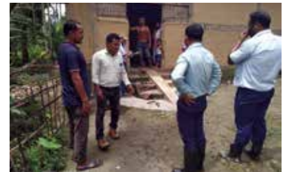
Survey by Committee constituted by District Administration on Assessment of Damage by the Blowout
