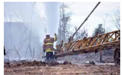
Removing of spool from Well Head at site on 22nd July 2020
