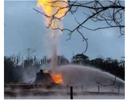
Debris Removal Job with Continuous Water Spraying
