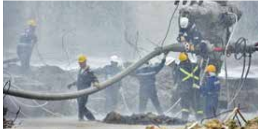
Preparation work before killing on 18th August 2020
